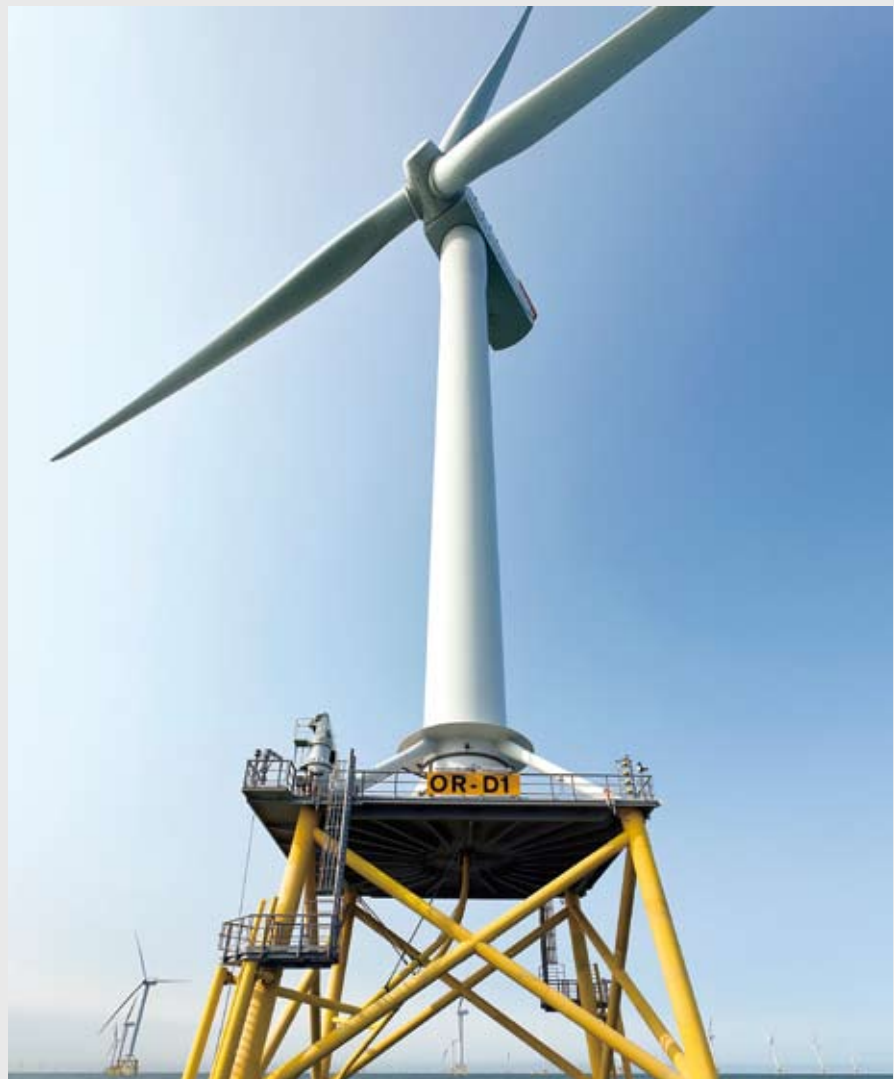
The OWEC Quattropod® design separates and optimises the piling and jacket installation process, resulting in reduced installation costs and faster project delivery
